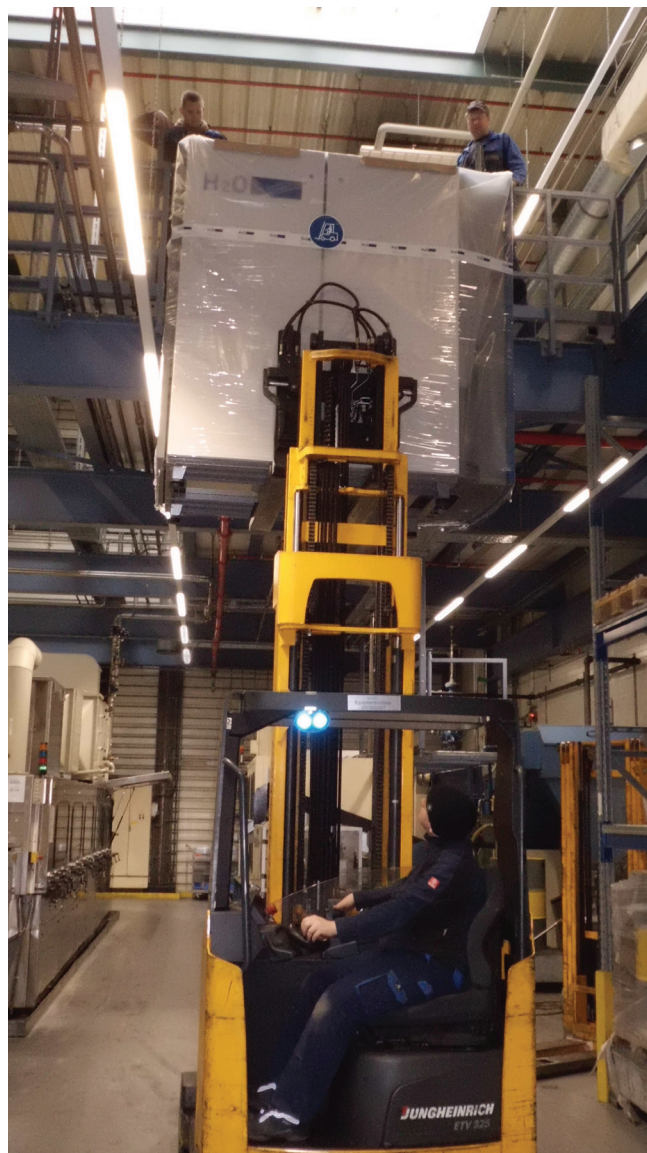
Complicated but ultimately successful forklift manoeuvring of the unit at a height of 5 m.
